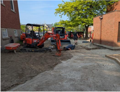
View of work in progress, near the entrance close to the Fellowship Lounge.
