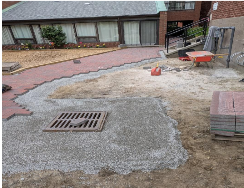
New interlocking stone, installation in progress.
